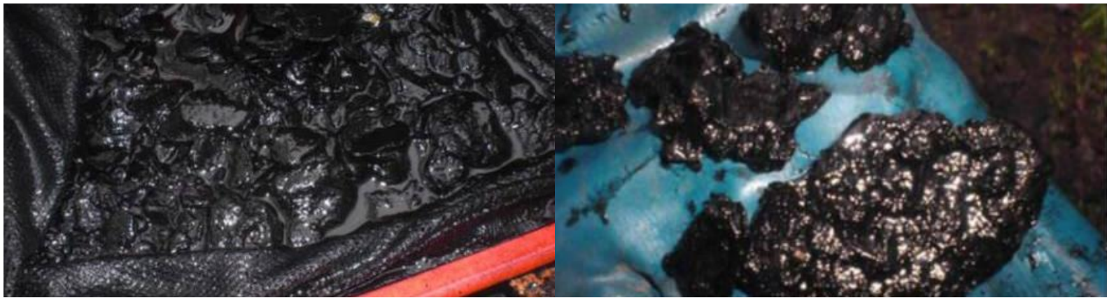
Figure 9: Aged grease deposits from wastewater pressure pipeline after complex impulse cleaning
